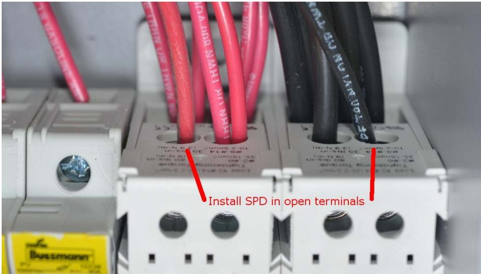
Image 5: SPD must be wired to their own dedicated terminals. This photo shows the six pre-wired PV+ wires and an example system consisting of five strings of PV circuits, hence only five PV- wires.
