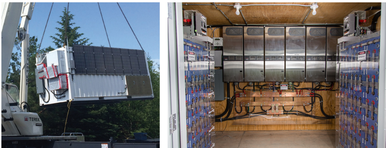
Figure 3: The Saskatchewan Research Council Hybrid Energy Container (HEC-60) at installation.
